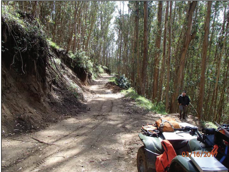
Photo 29 (Site #11): View of the hydrologically connected left road approach to landslide Site #11. Long reaches of concentrated road runoff have eroded a gully down the outboard fillslope and induced a failure.
