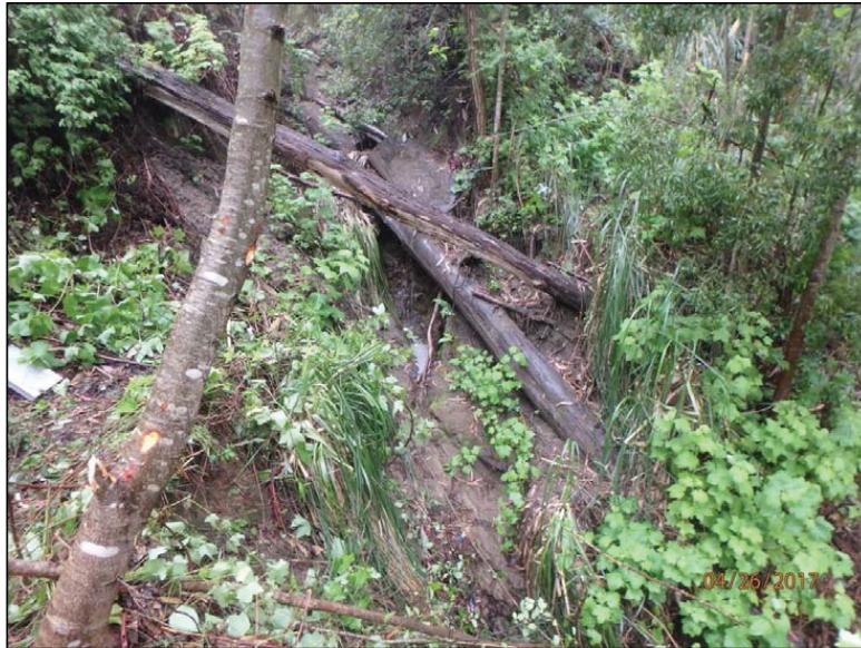
Photo 19 (Site #41): View looking upstream at a washed out fill crossing on a near origin Class III stream downslope from residential area on Santa Maria Avenue. This view of the scoured stream channel was taken from the outboard edge of road at Site #41.
