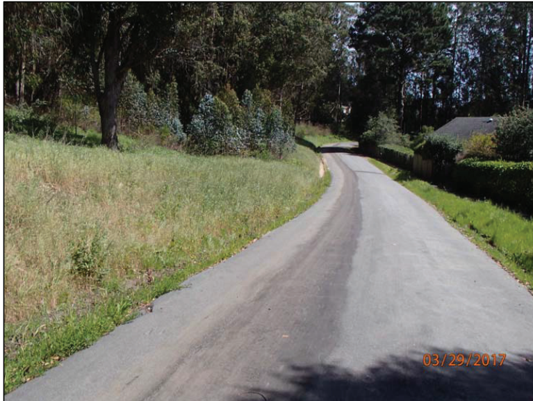
Photo 37 (Urban Drainage Interface – AOC 3): View of the urban drainage interface located on Moro Ave, (AOC 3, Map 2). Flow is conveyed down the inboard ditch for ~325' to a ditch relief culvert at the intersection of Santiago Ave. and Moro Ave. The crowned road surface keeps the majority of the stream flow on the inboard edge of the road.
