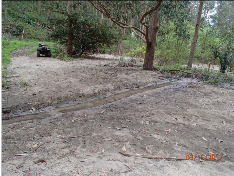
Photo 9 (Site #2): View of stream crossing through this shallow sediment filled pond. Stream sediment transport has deposited a large volume of fine sediment in this old pond, inundating the pond and trail.
