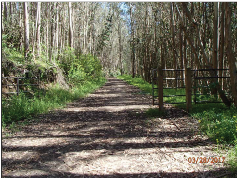
Photo 2 (Miranda East Fire Road): View of the existing road conditions on the Miranda East Fire Road at Gate 4 as shown on Map 2.
