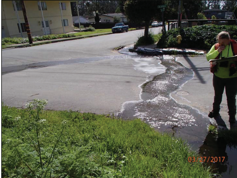
Photo 35 (Urban Drainage Interface - AOC 2): View of uncontrolled Class II stream flow exiting the Park at Santa Maria Avenue (AOC2, Map 2). Combined flow from the stream and road surface runoff travel down Santa Maria Ave. The majority of the Park's drainage area evacuates the Property into the residential area downstream at this location.
