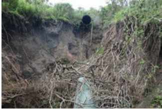
Erosion repair example
