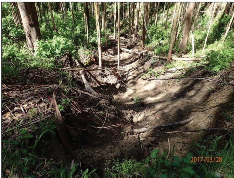
Photo 26 (Site #31): View of an outboard fill failure at Site #31 on the Vista Point Trail. Concentrated road run off had saturated the steep outboard fill and subsequently destabilized the fillslope leading to failure.
