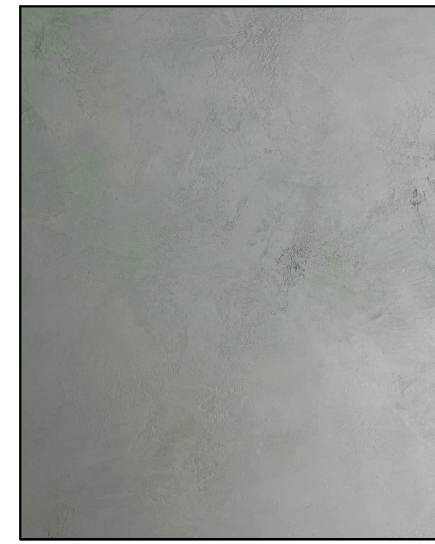
EXTERIOR: PLASTER - CEMENT SAGE
