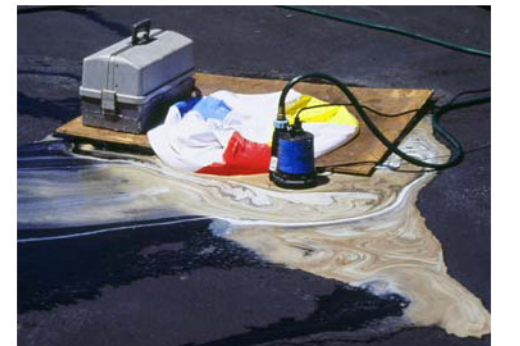
Storm drain inlet is blocked to prevent prohibited discharge. The water must be pumped and disposed of properly.
