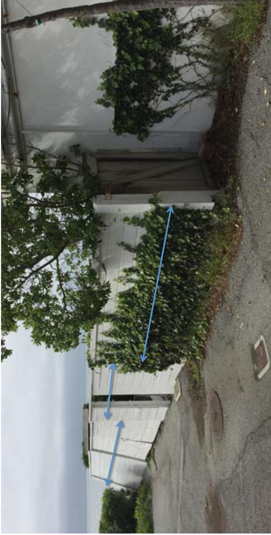
South fence section and double gates proposed for removal have failed and are leaning against the Cypress behind.
